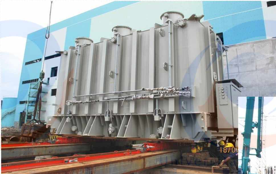
377 Ton Transformer at Cirebon Power Plant
