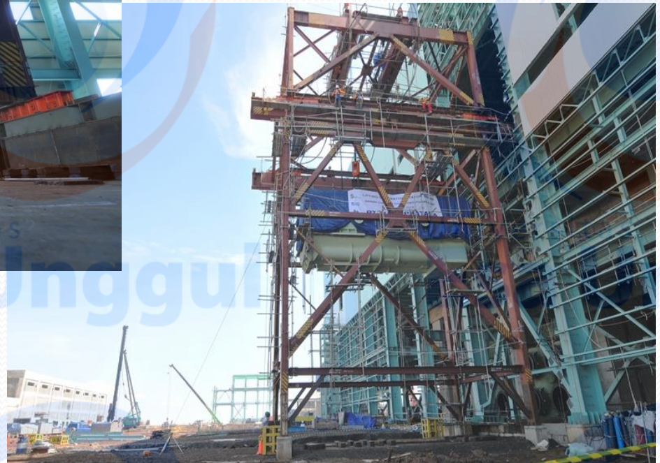
285 Ton Generator Stator at Cirebon Power Plant
